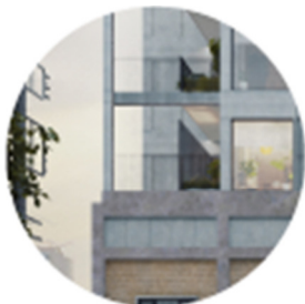
3. Proposed concrete framing with galvanised metal cladding
