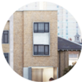
1. Existing concrete details around windows
